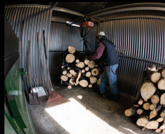
The smoke coming out of the chimney is from excessively dry wood not recommended by the manufacturer (or Dick). But even with the wrong wood, the system is virtually smokeless after the initial 5-15 minute start-up cycle.
