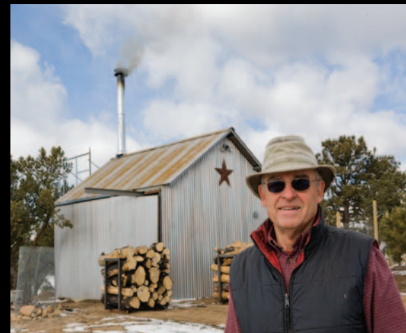
Wood-heating pioneer Dick Cook designed and built the boiler shed and very convenient wood handling system for his 300,000 BTU/hr boiler. Dick has been testing a variety of wood drynesses and species.
