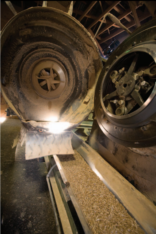
Pellet mill open for cleaning
