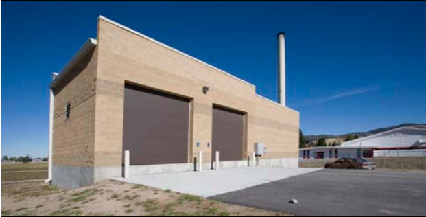
Wood-chip boiler building that heats the Darby School, the first Fuels for Schools project in Montana.
